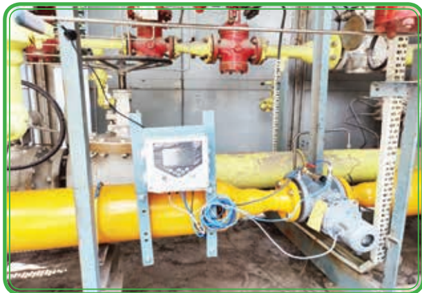
AMR Meter installed in DRS
