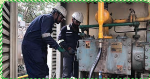
Compressor Maintenance in progress.
