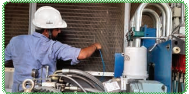
Booster Gas Cooler Cleaning Work
